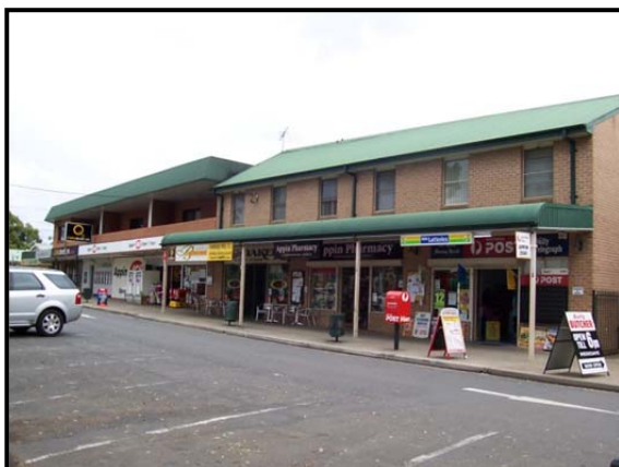
Photo 13: Appin Local Shops.
