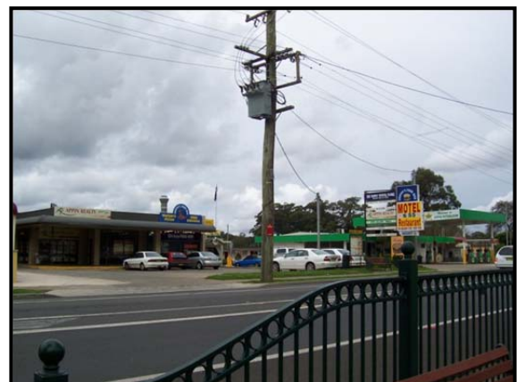
Photo 14: Appin Local shops.
